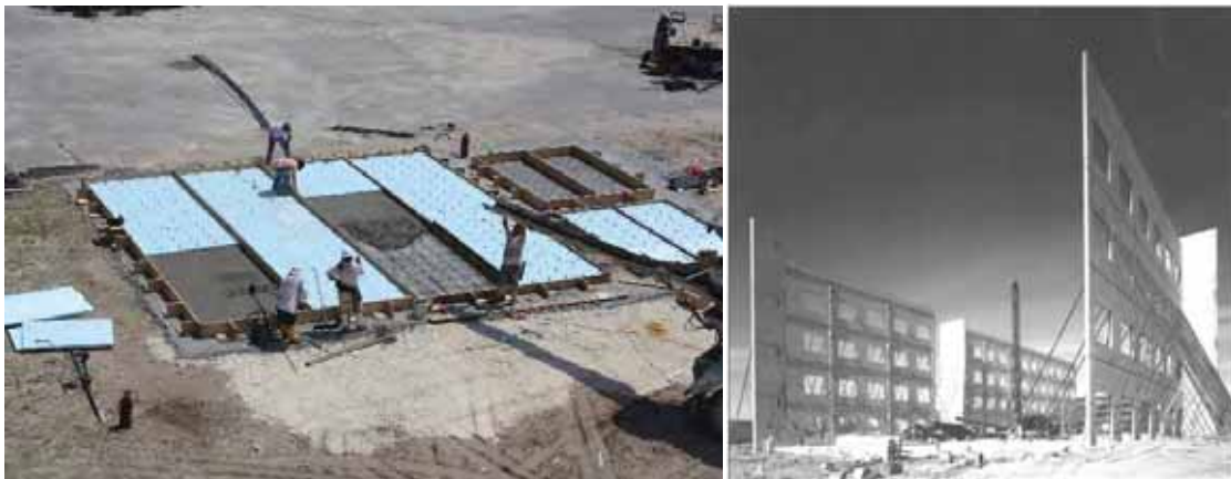
Figure 2. Tilt-up Concrete Sandwich Wall Construction [TCA 2006]
