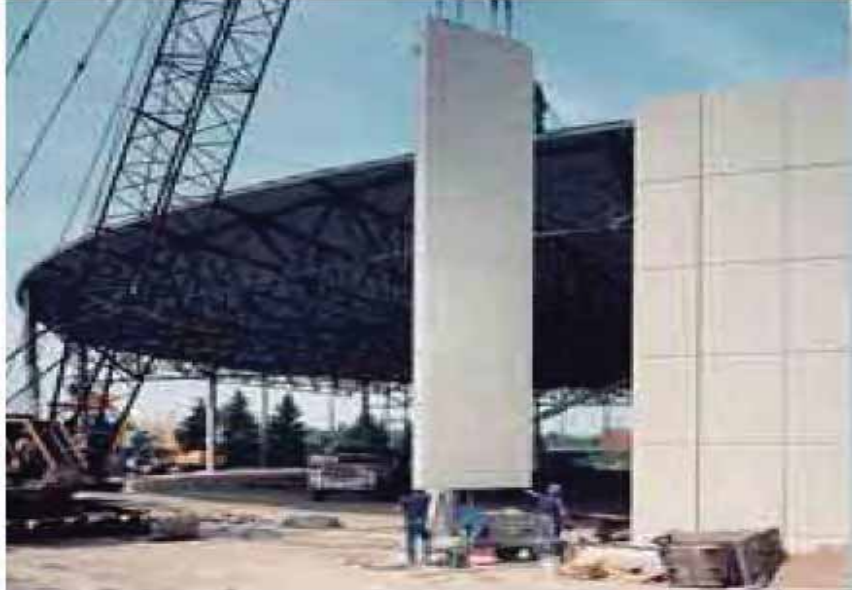
Figure 3. Prestressed Concrete Sandwich Wall Construction [PCI 1997]
